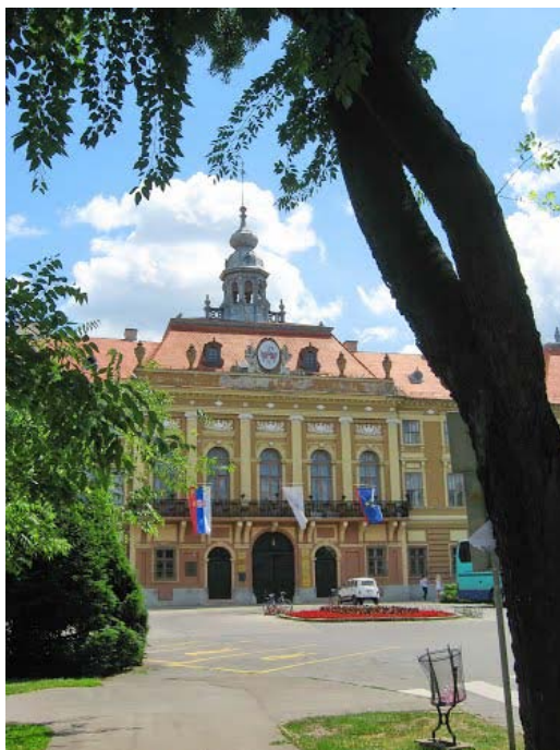
Figure. The town hall in old city centre of Sombor [21]
