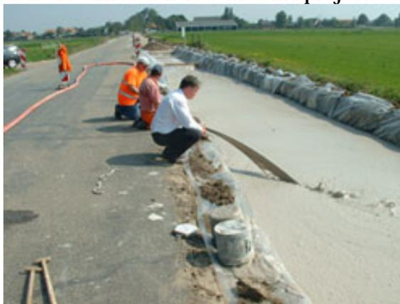
Figure 1: Road in Holland is being widened and foamed concrete was used for the road sub-base
